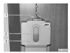
Fig. 196 Compensator reservoir hotwater heater
